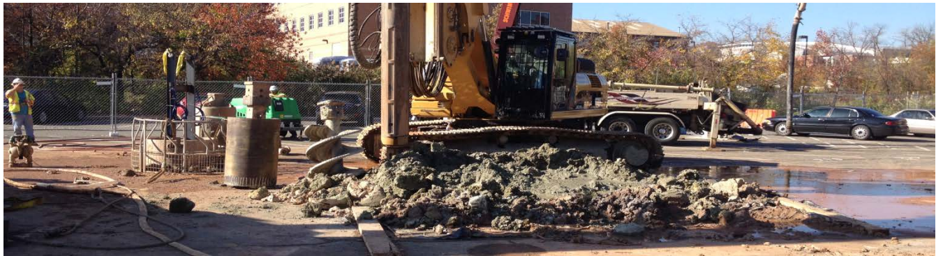
Drilled shaft excavation.
